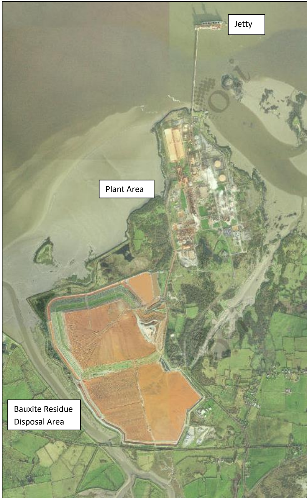
Figure 2.2. Aerial View of Aughinish Alumina Limited (Source: Geohive Aerial Premium Map)
