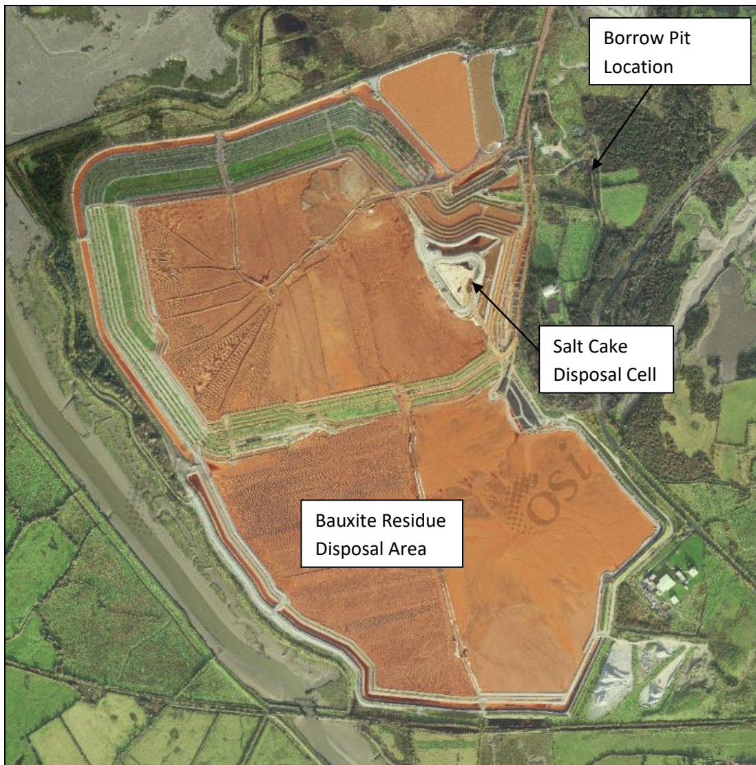
Figure 3.1: Aerial View of part of Aughinish Alumina Site – BRDA (Source: Geohive Aerial Premium Map).
