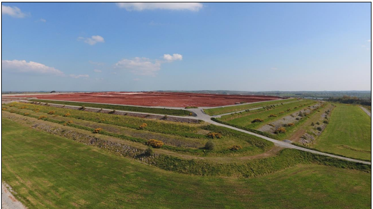
Figure 3.3: Image of BRDA illustrating Upstream Construction Method
